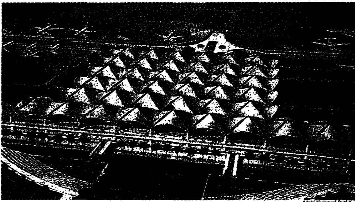
Main Terminal Building
